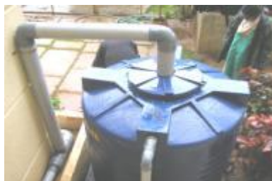
Rain barrel with online filter at Adarsh Apartments
