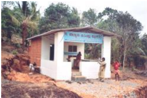
Cashew processing centre
