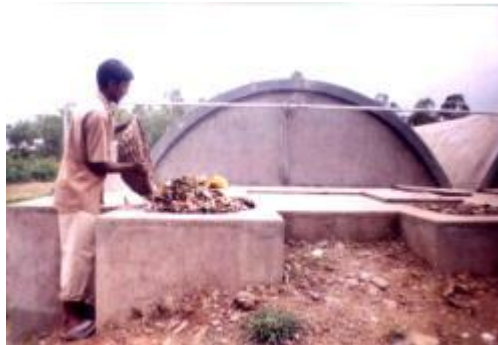
Organic municipal waste being fed into bioreactor during commissioning
