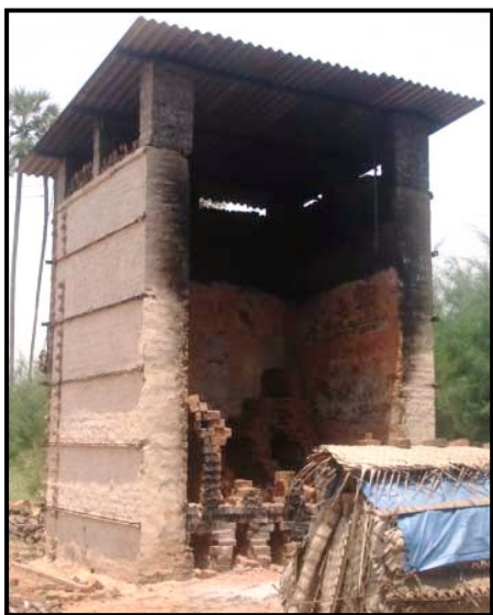
Low capacity brick kiln
