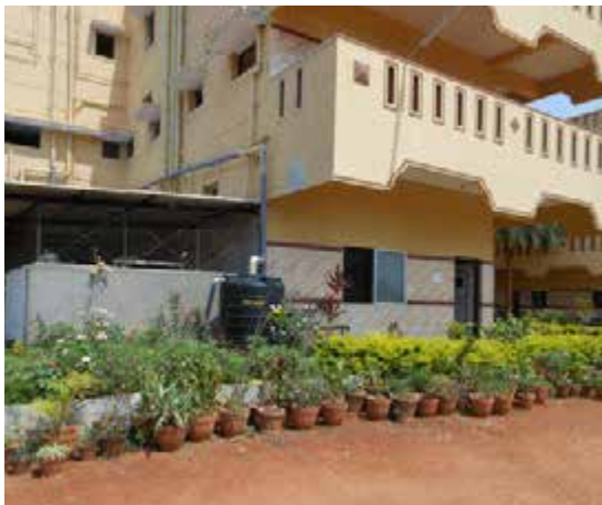
Rooftop rainwater collecting system
