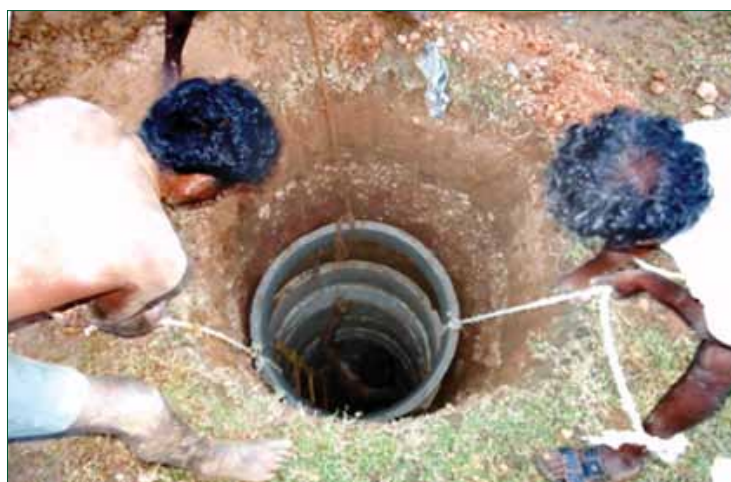
Figure 2: Recharge well being constructed
