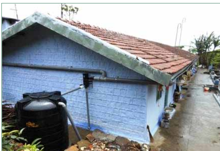
Figure 11: Tea estate labour colony- Roof top rain water harvesting
