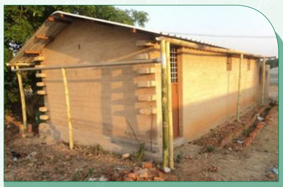
Figure 4: Bamboo based Roof top rain water harvesting system
