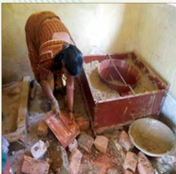
Figure 6: Construction of low cost mid day meal cook stove
