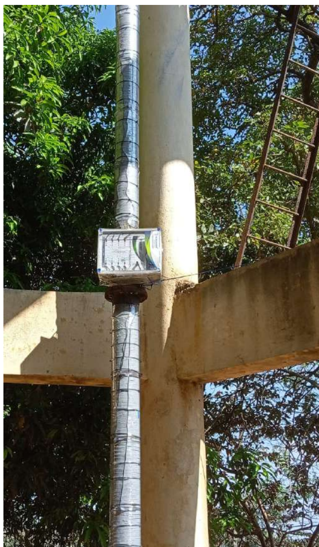
Water softener installed on campus
