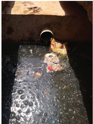
Storm water drains mixed with black water
