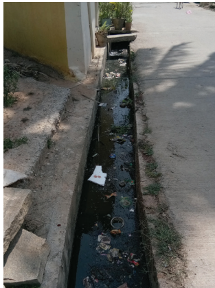
Clogged storm water drains in the city
