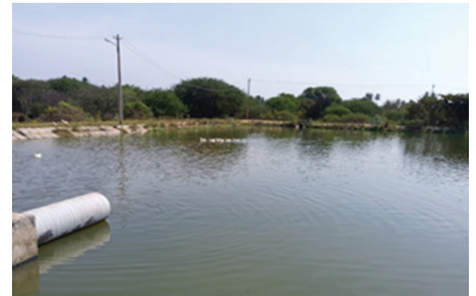
Oxidation pond at the STP
