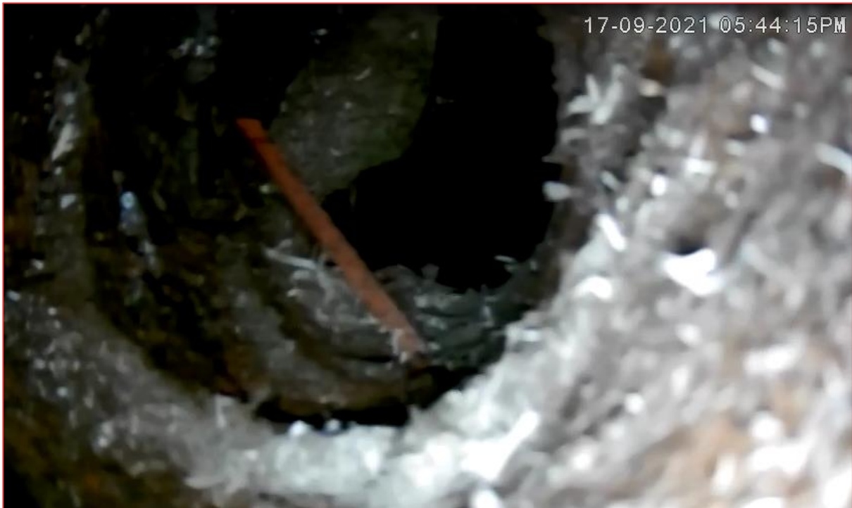
CASING IS IN DAMAGE CONDITION
