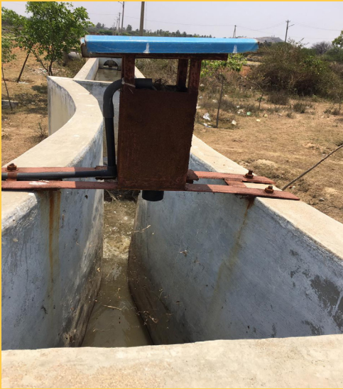
Dysfunctional flowmeter
