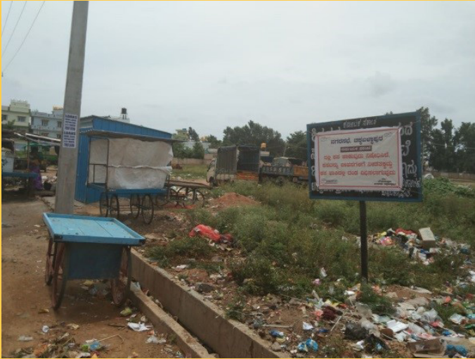
Figure 6.5 Dumping of solid waste in drains and open fields.
