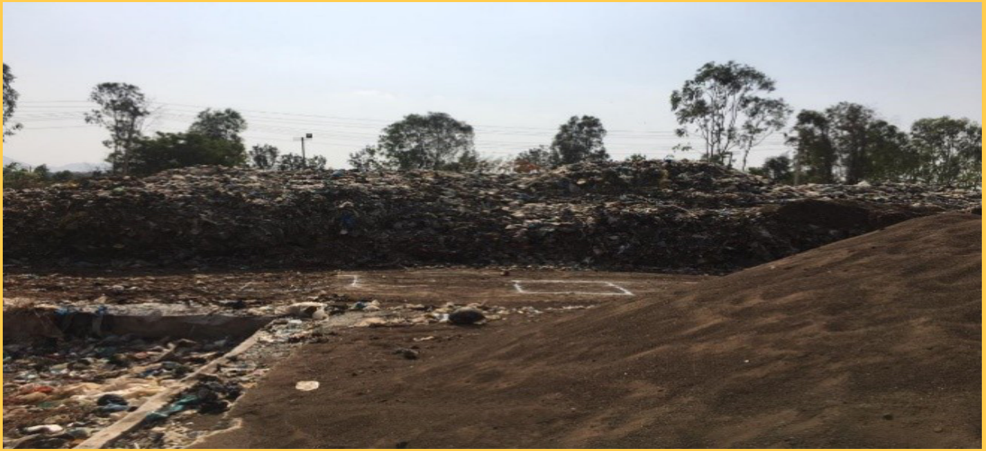
Figure 6.3 Legacy waste at dump site, Chikkaballapur
